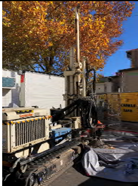
PHOTOGRAPH 28: BOREHOLE BH01 INSTALLATION
